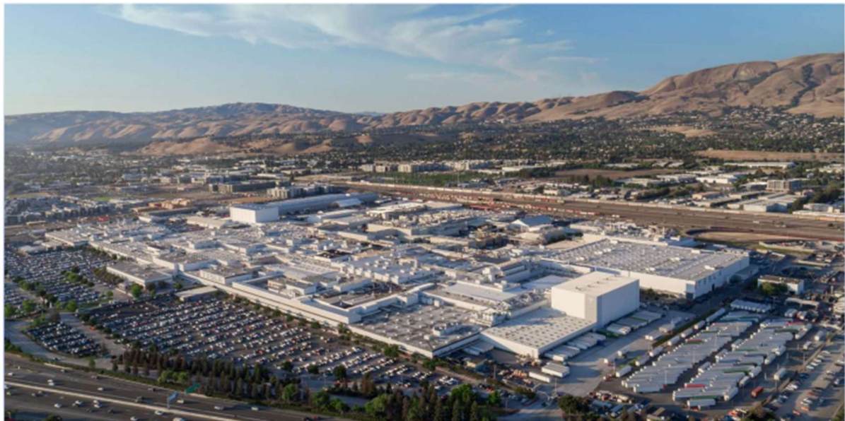
Tesla's 5.3 million square foot factory in Fremont, California.
